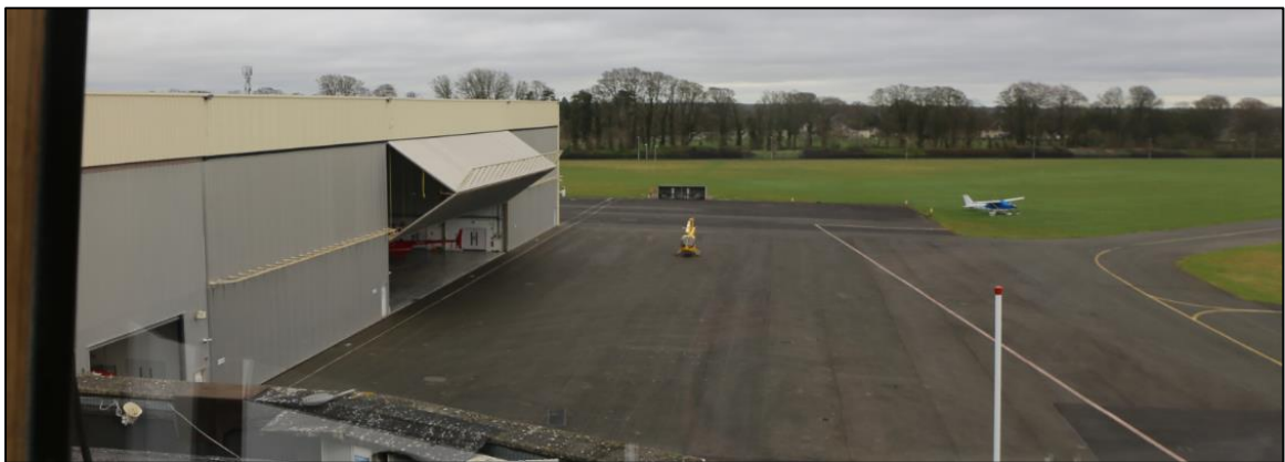
Photo No. 4: View from the control tower of the south apron
