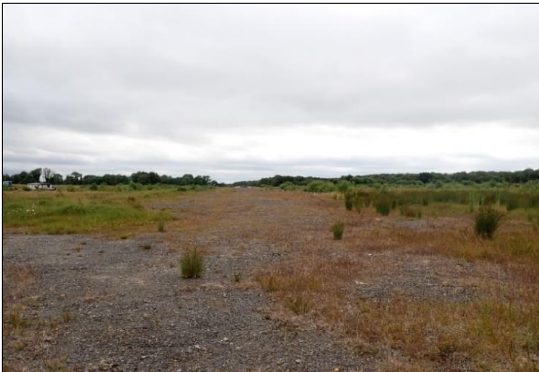
Photo No. 6: View of RWY 24
