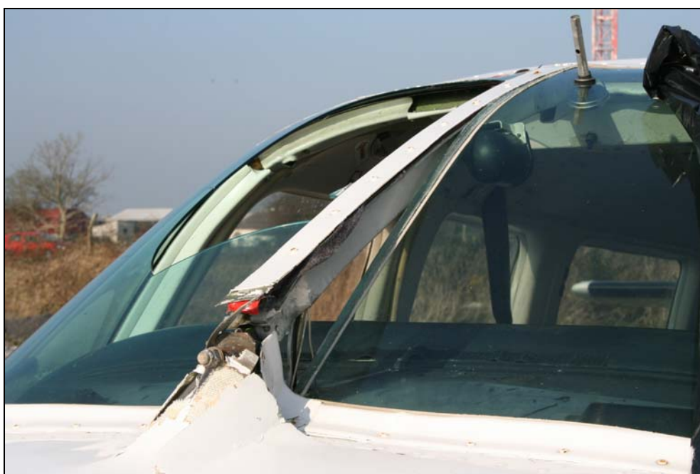
Photo No. 1: Showing apex of 'A' frame protruding 4 inches above fuselage nose and the severed windscreen support.
