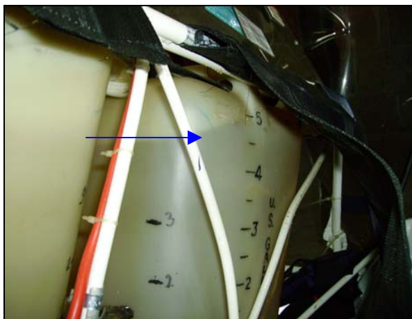
Photo No. 2: Left Tank – approx. 4 ½ USG
