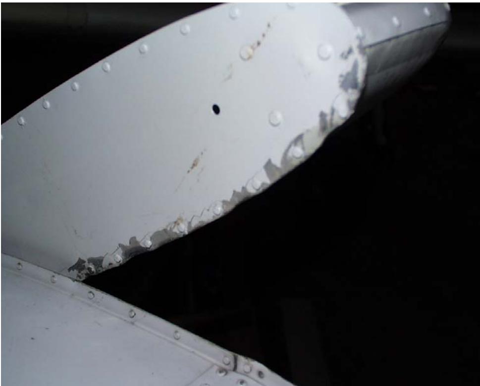
Photo No 2. Damage resulting from cables running across the lower surface edge of the port mass balance horn of the elevator
